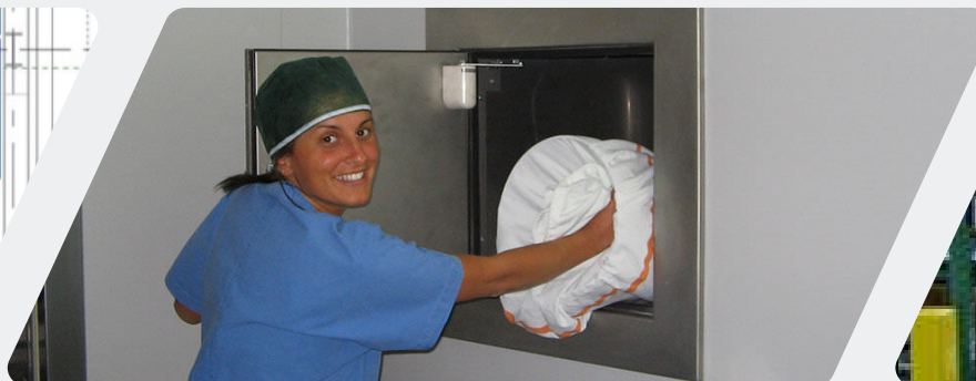
Pneumatic Chute Systems
